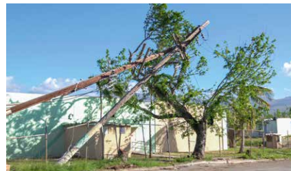
Maria knocked down 80 percent of Puerto Rico's utility poles and all transmission lines, resulting in the loss of power to essentially all of the island's 3.4 million residents.
