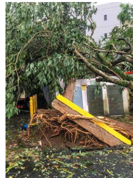
A fallen tree outside the Los Paseos Dialysis Clinic narrowly missed the generator.
